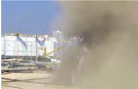
CONVENTIONAL ABRASIVES CAN CREATE EXCESS DUST
