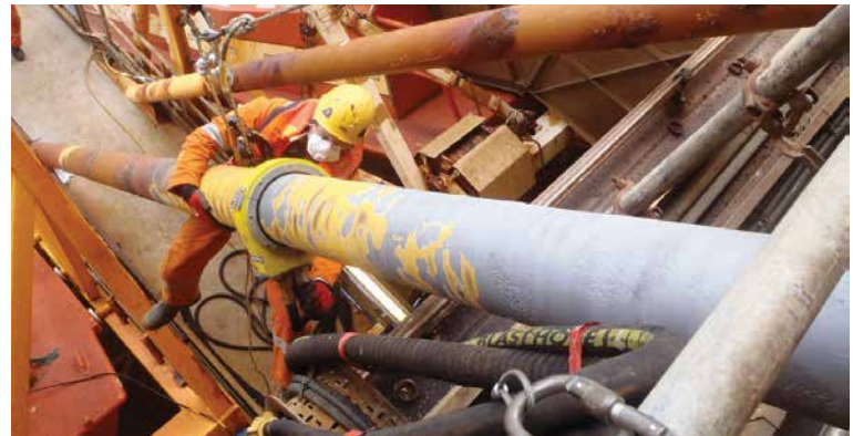
This worker is blasting a 8" pipe on an off-shore oil platform. He is using a rope access system to save the cost of scaffold and containment.
