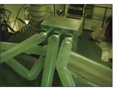
Fig. 8: Closed loop dehumidification system with even distribution set up
