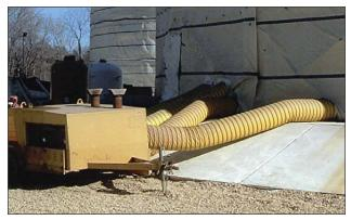
*Fig. 4: Amount of heat required is significantly reduced when using 0.25 inches of insulation on the tank.*
