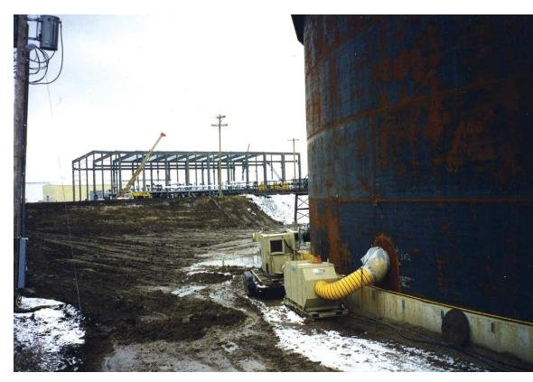
Fig. 1: All heaters discussed here are placed outside the tank because of size constraints, fuel fumes, and other safety issues.
