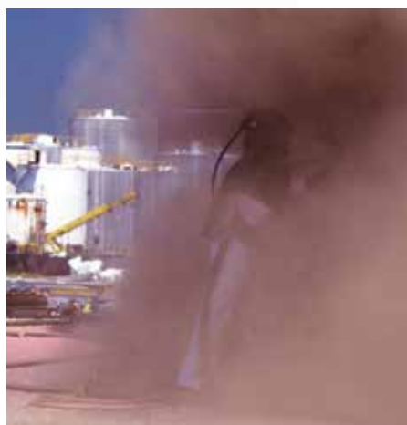
Conventional abrasives can create excessive dust.
