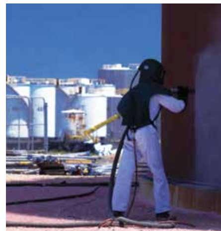
Blasting with GMA Garnet is much more neighborly.
